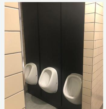
Our made to measure metal framed washroom panelling system, Frameduct, was specified in matching Noir HPL for the WCs and urinals. With Frameduct, all duct space is concealed and can be accessed by opening the secure access panels that are on 90° linear bearing hinges - this makes for simple ongoing maintenance.
